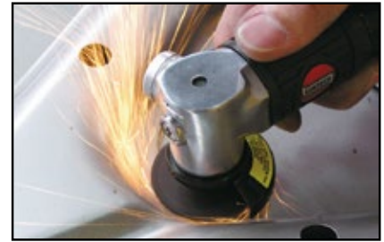
▲ Operation of Cutting Metal Plate
