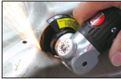
▲ Operation of Cutting Metal Plate
