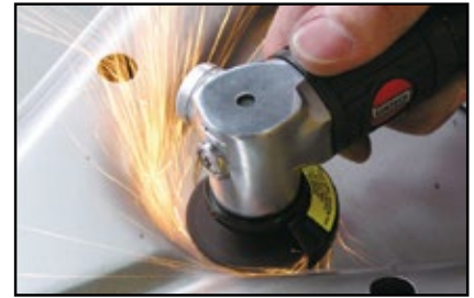
▲ Operation of Cutting Metal Plate
