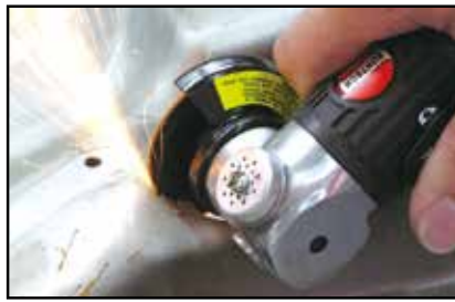
▲ Operation of Cutting Metal Plate
